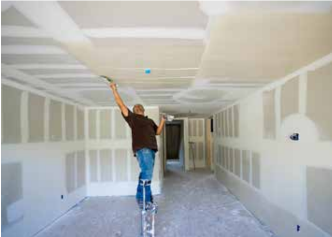
Figure 1. Illustrates the use of joint compound to finish interior walls and ceilings.
